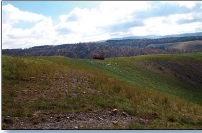
Figure 2. Red River Coal Company revegetated and regraded mined areas to reduce erosion and restore original contours on mined areas.
