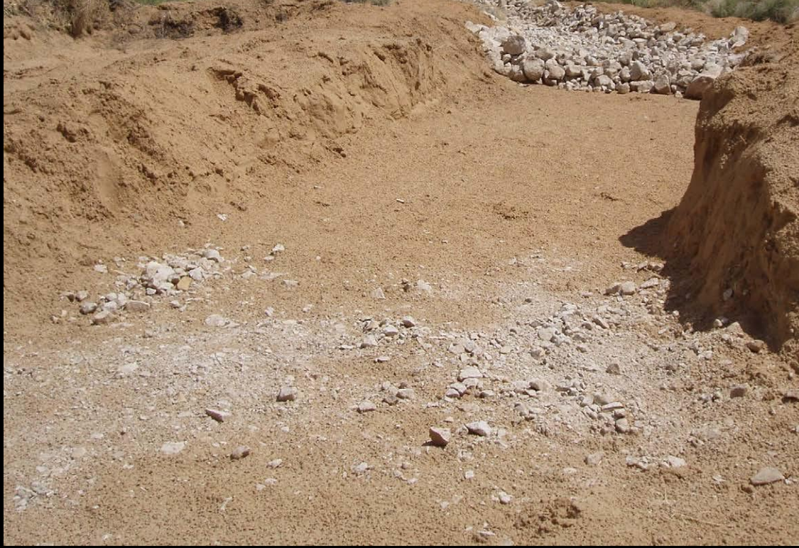
Installation of a rock water bar will help slow water flow and divert water away from the spring.
