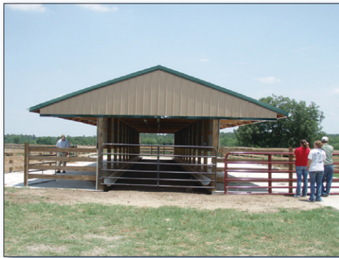
Figure 4. To address the runoff from the heavy use feeding area, the landowner built a structure that keeps the cows dry during feeding and allows for easy clean up of manure.
