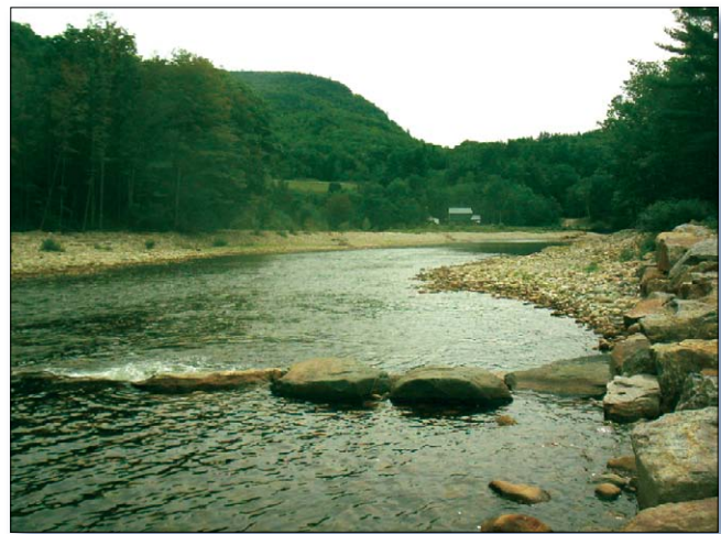
Figure 1. A porous rock weir helps to stabilize the restored section of the Pemigewasset River.
