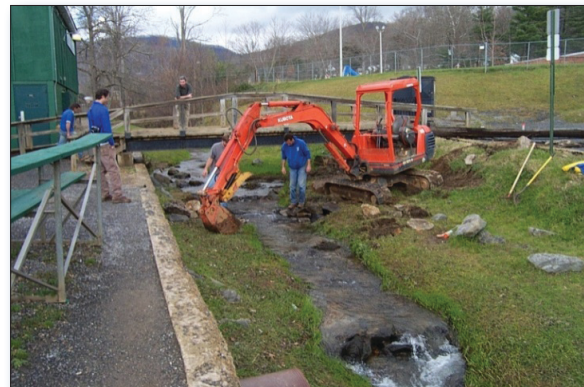
Figure 1. Project partners restored streambanks along a developed portion of Haw Creek, a tributary of the Swannanoa River.
