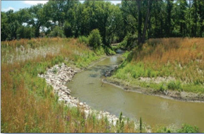
Figure 2. Partners installed numerous BMPs, including this streambank protection project on Dows Creek.
