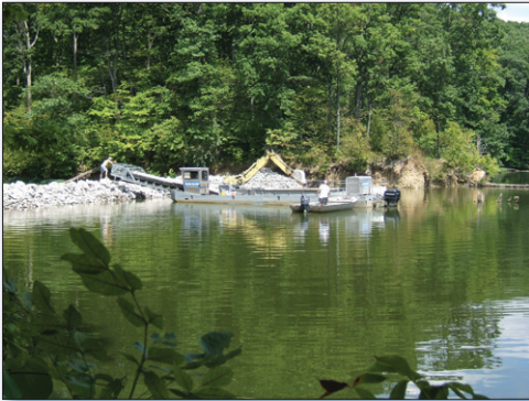
Figure 3. The city installed an in-lake sediment detention basin; note the difference in water clarity between the upstream side (left) and lake side (right).
