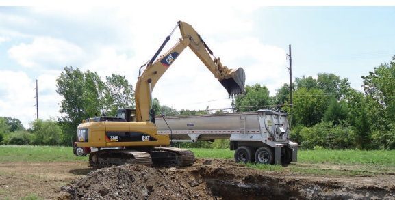
A backhoe is removing asbestos-containing materials from the site.
