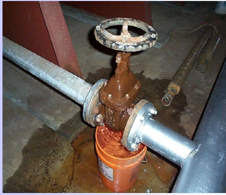
Leaking valve
