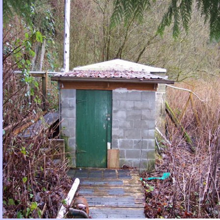
Booster station with above ground piping Credit: Rural Community Assistance Corporation
