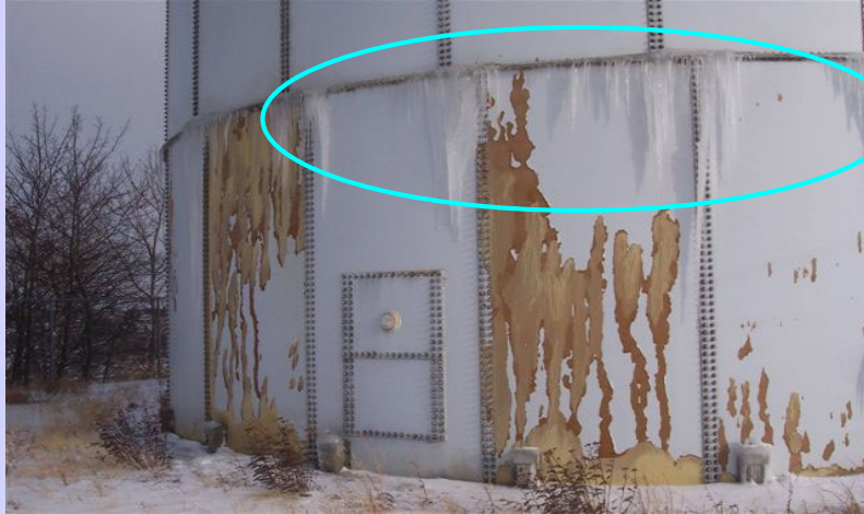
Leaking reservoir
