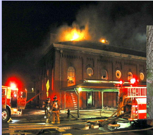
Fire at DC's historic Eastern Market Credit: Arthur Delaney, Washington City Paper
