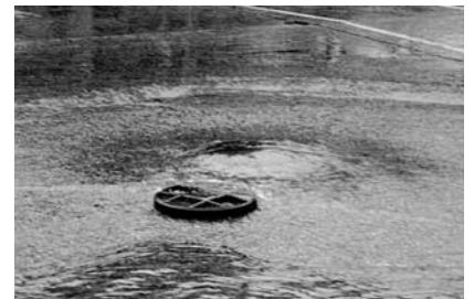
SSOs include untreated discharges from SSSs that reach waters of the United States, as well as overflows out of manholes and onto city streets, sidewalks, and other terrestrial locations.
