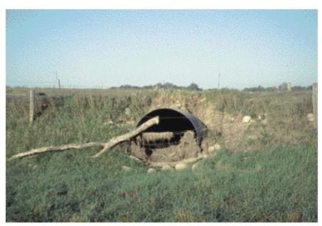
This road could fail if debris is not cleared before the next heavy rain.
