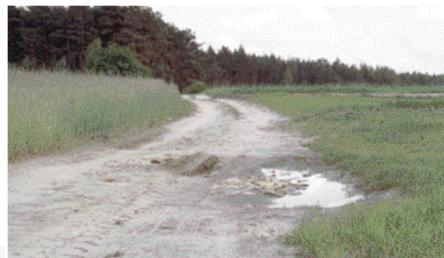
This road located in Poland has very poor cross section.Consequently, drainage and overall driving conditions are bad. (Courtesy of Mary O'Neill, Office of Remote Sensing, South Dakota State University, USA)
