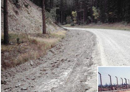
A nicely reshaped ditch that meets the shoulder line of the road and allows good drainage.
