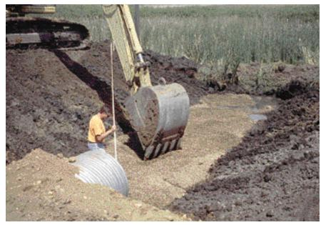
New culverts installed well and at correct elevation are essential for carrying water under a road.A reasonable maintenance schedule is required to keep them functioning well.
