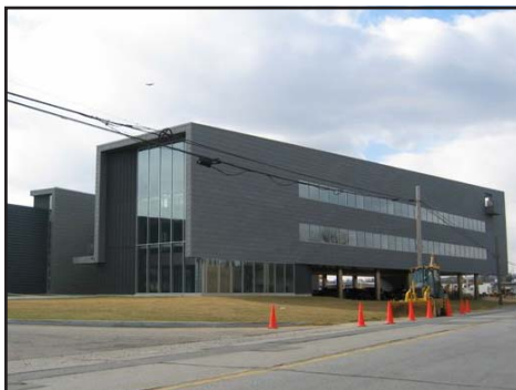
The completed Buccini/Pollin headquarters.
