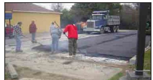
Site remediation in progress.
