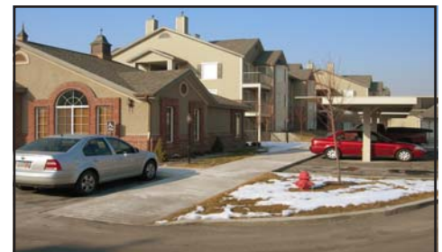
View of the new clubhouse/office and new apartment buildings.
