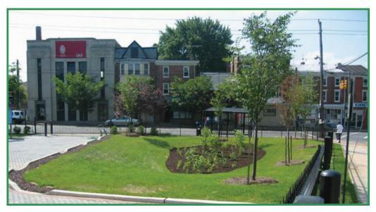
A bioswale in Wilmington, Delaware, designed to absorb and retain stormwater runoff.
