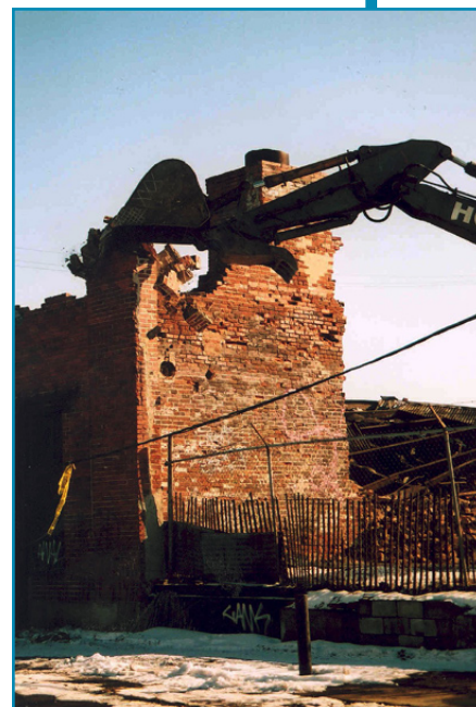
Demolition of structures underway on the former SPECO Kelsey-Hayes site.
