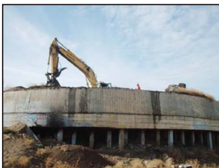
Construction underway at Kendall Yards.
