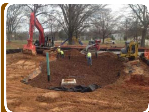
Installing green infrastructure in the Proctor Creek neighborhood of Atlanta, GA.
