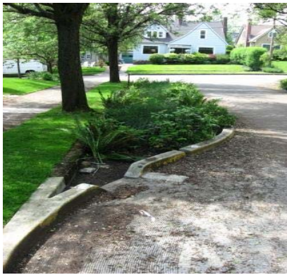
Vegetated curb extensions used in Portland, Oregon, to decrease stormwater runoff. (EPA photo)
