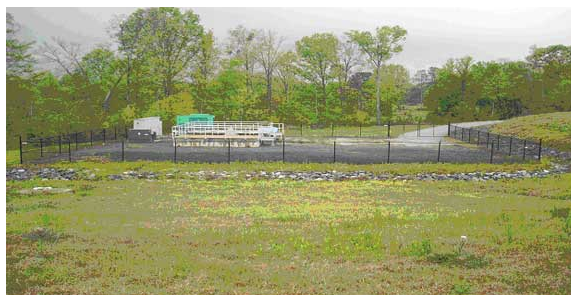
City of Flowood pump station. (EPA OIG photo)
