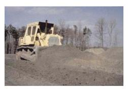
Spreading and compacting fly ash structural fill. (EPA photo)
