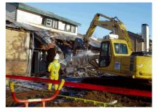
An example of the beginning stage of the Alternative Asbestos Control Method process. (EPA photo)
