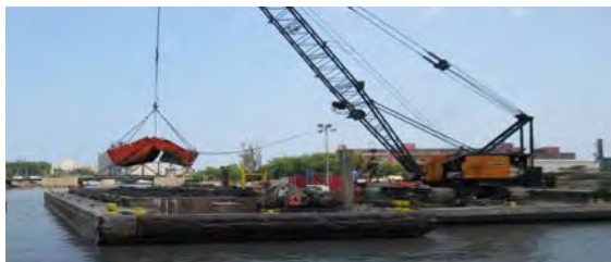
Equipment cleaning sediment at Kinnickinnic River site, Wisconsin. (EPA photo)
