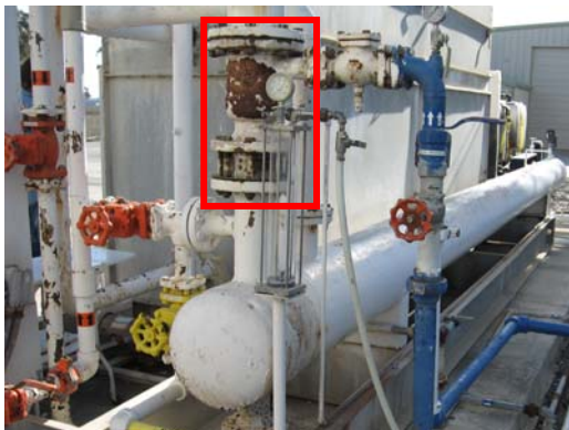
Heat exchanger used to heat anhydrous ammonia before it flows to a reactor to produce a fertilizer product at a risk management program facility. The highlighted area shows visible corrosion. (EPA photo)
