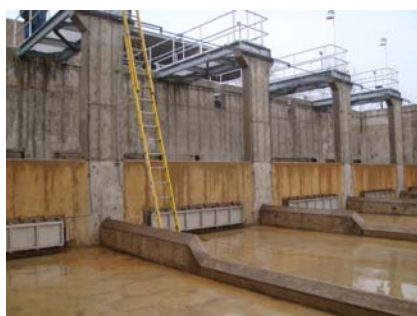
Flushing gates at the Goshen Combined Sewer Overflow Detention Facility. (EPA OIG photo)
