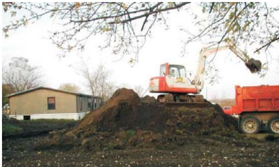
Heavy equipment removing contaminated residential soil in Cherryvale, Kansas. (EPA photo)
