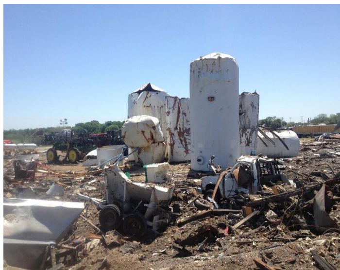
Damaged volumetric tanks and equipment at the Adair Grain Inc. Fertilizer Plant in West, Texas. (EPA photo)
