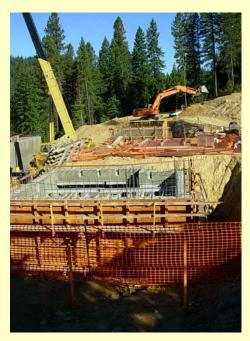
Above: Construction activity on the water pump station and neutralization and backwash equalization pump stations for the Central Shoshone County Water District project. (EPA photo)
