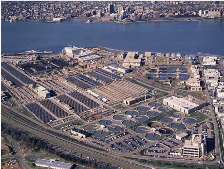
The Blue Plains Wastewater Treatment Plant in Washington, DC, a major treatment facility within the Chesapeake Bay watershed (photo courtesy District of Columbia Water and Sewer Authority).
