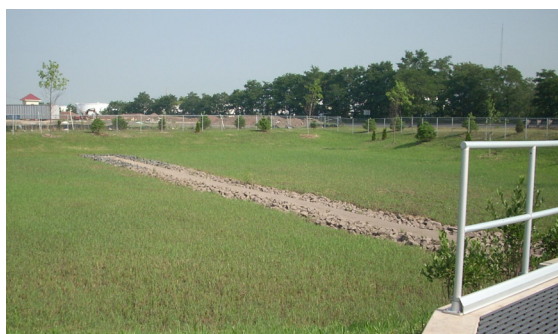
Stormwater holding pond at the Hill District Stormwater Pumping Station in Carteret (EPA OIG photo).
