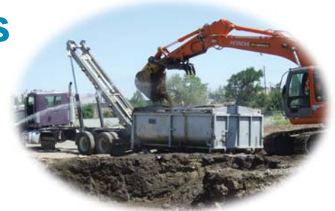
Soil remediation underway.
