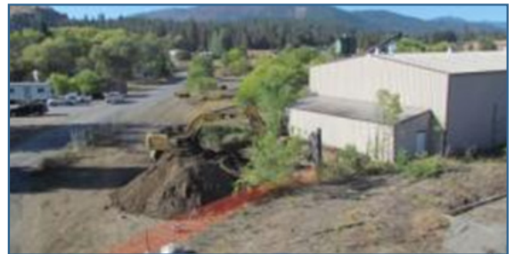
The former Inchelium Wood Treatment Facility.
