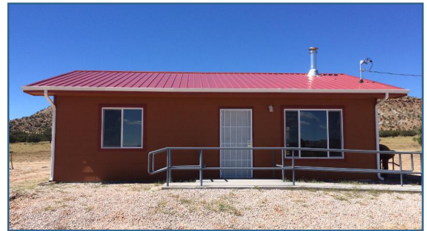
Navajo residential house after cleanup action.
