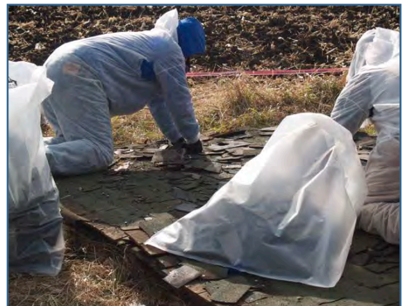
Asbestos Cleanup Activities on the Flandreau Santee Sioux Reservation.
