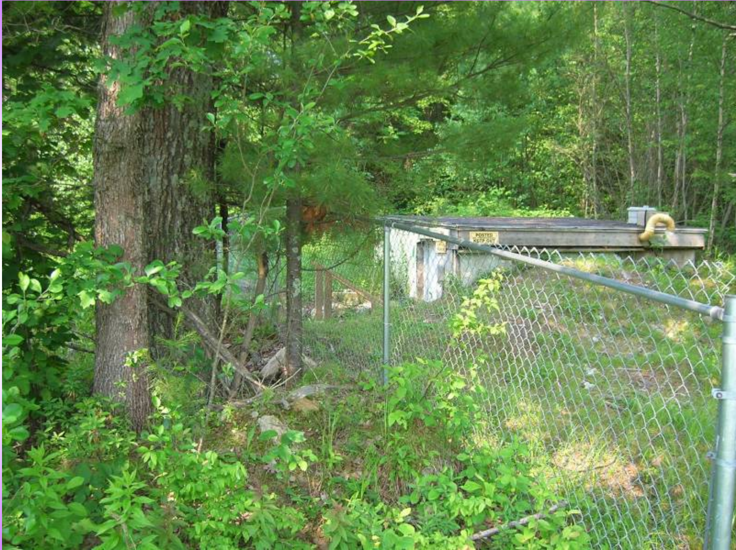
Well House and Treatment - Pelham, NH
