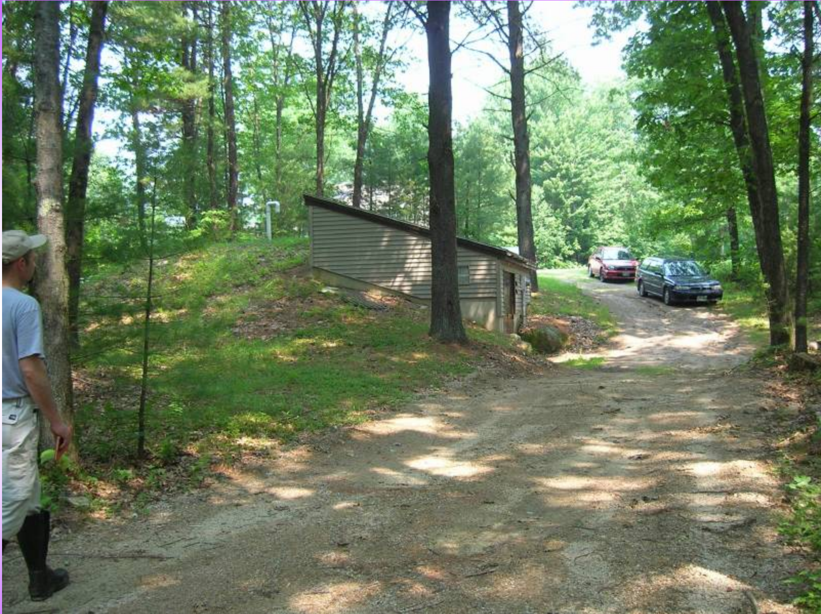
Well House and Treatment - Bedford, NH
