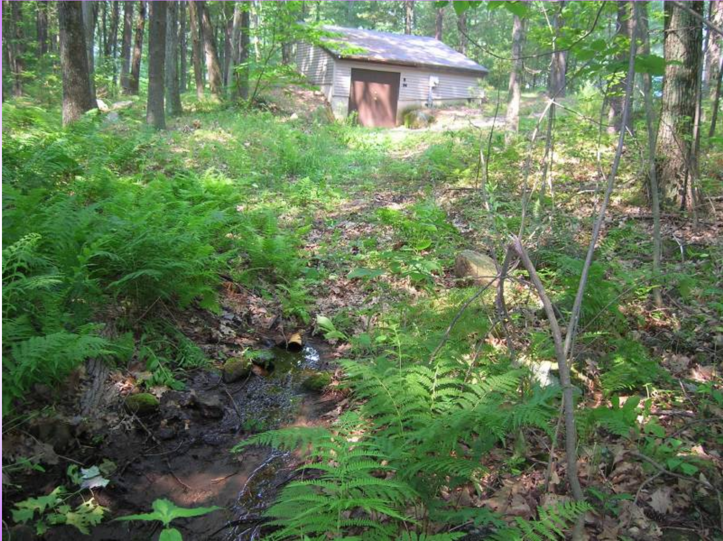
Well House and Discharge Pit - Bedford, NH
