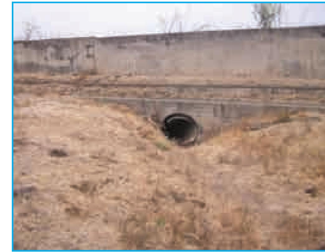
A dysfunctional culvert and retaining wall carry a tributary to Walters Creek.
