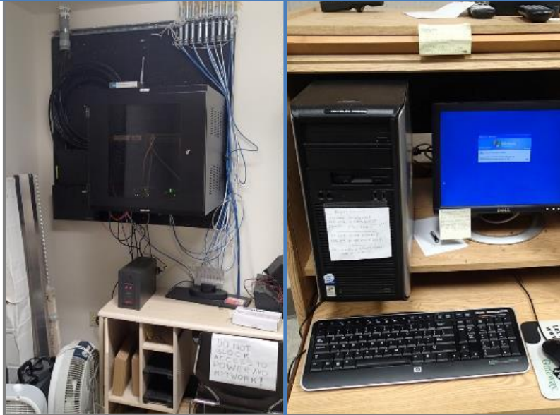
Figure 3. The Electronics that Remained in the House during Fumigation
