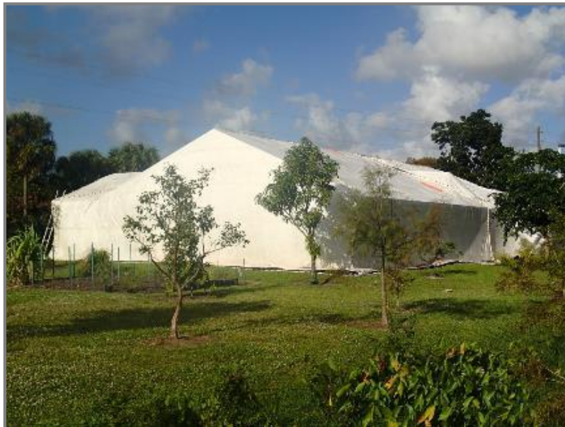
Figure 9. In Preparation to Fumigate, the House was Sealed with Two Tarps
