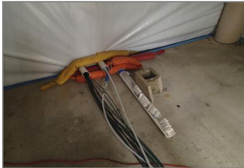
Figure 12. Monitoring Lines, Shooting Lines and Coupon Slide Inserted Between the Skirt and Apron (View from Inside House)
