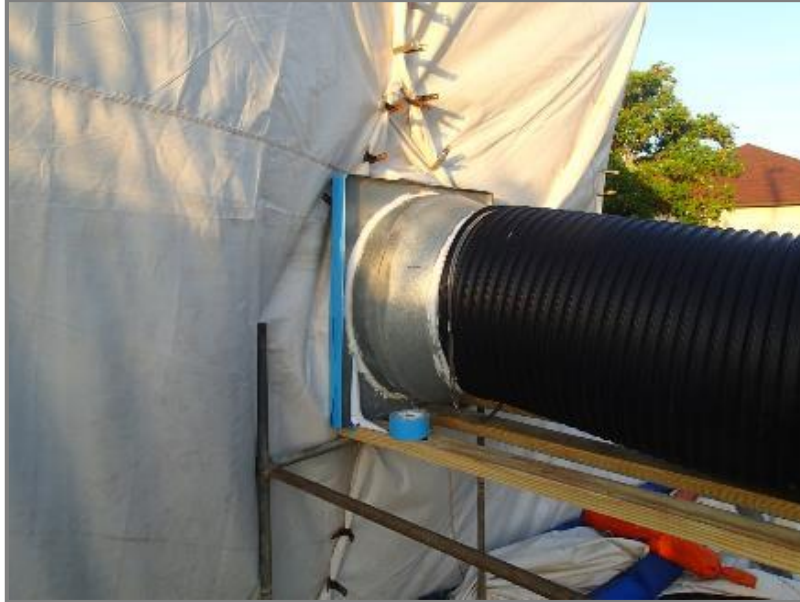
Figure 11. Flange of Carbon Scrubber Exhaust Port Joined to Tarp at a Seam
