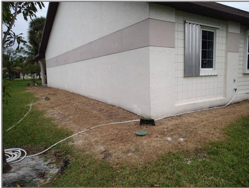
Figure 42. Grass Kill as a Result of MB Diffusion Through the Ground-seal Apron.
