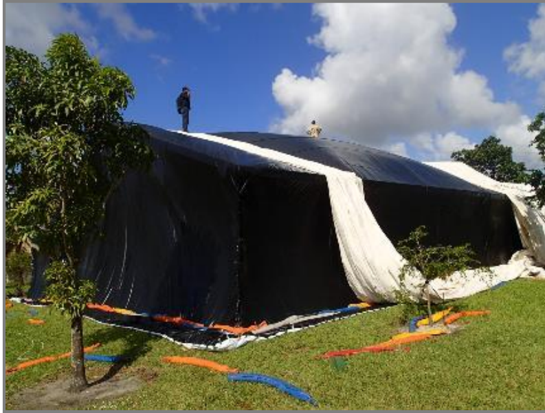
Figure 8. Second Tarp (White) Positioned Over Black EVOH Tarp
