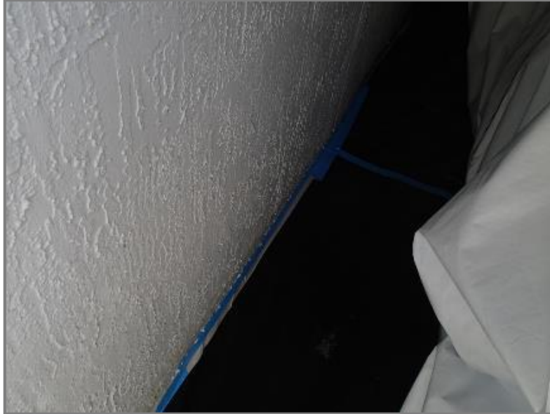
Figure 6. View of the Skirt of EVOH Tarp Dropped to the Apron on the Ground
