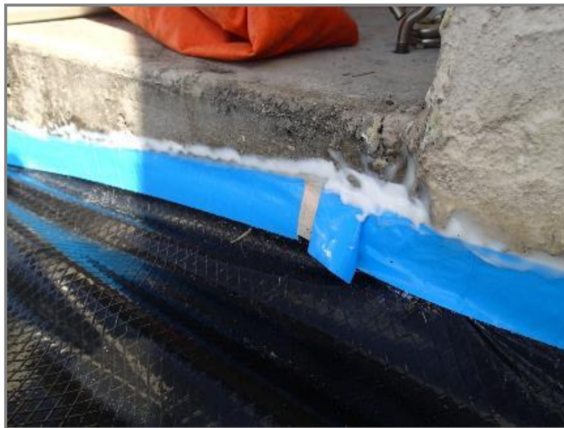
Figure 5. Attachment of Tarp Apron to Foundation of House with Tape and Caulk
