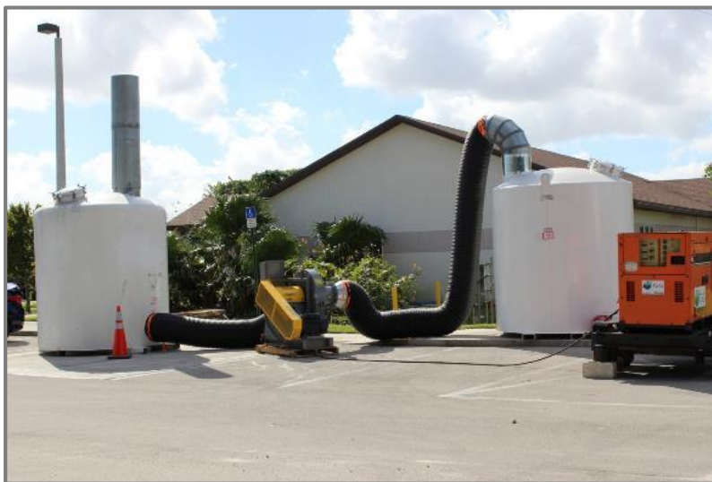
Figure 21. Activated Carbon Scrubber Installed at the House
