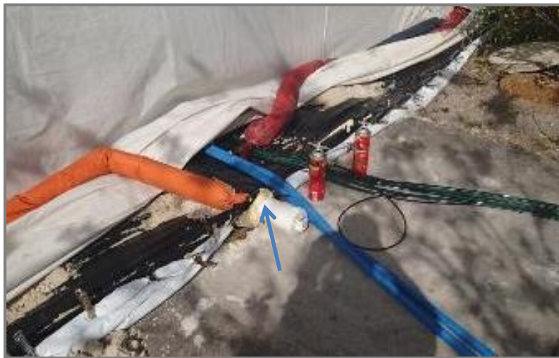
Figure 14. PVC Pipe Voids and Pipe Chases Filled with Expanding Polyurethane Foam.
