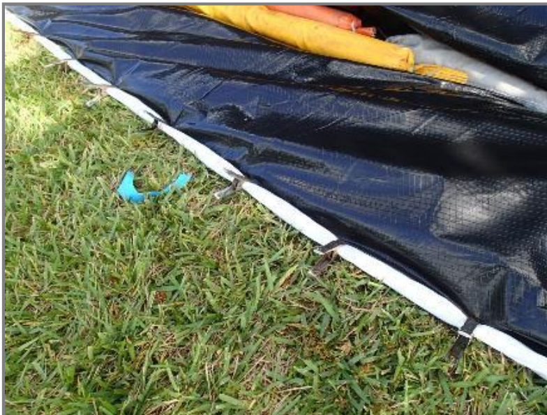
Figure 7. To Seal, the Skirt and Tarp Covering the House Were Rolled and Clamped at Edges and Weighed Down with Sand Snakes
