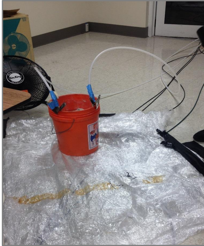
Figure 13. Bucket Release Point of Fumigant Inside House with Mixing Fan
