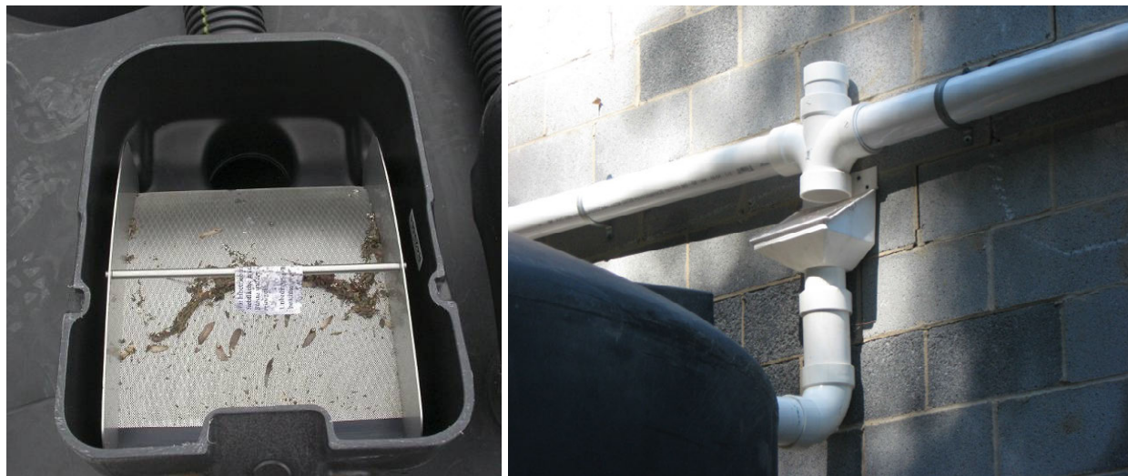
Figure C-5. Self-cleaning inlet filters.
