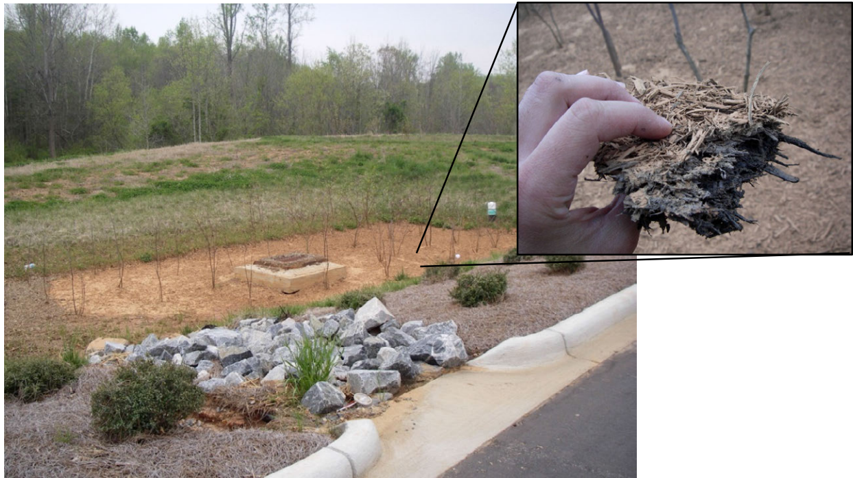
Figure 5-11. Example of a bioretention area installed before permanent site stabilization with the inset photo showing the clay layer clogging the mulch surface.
