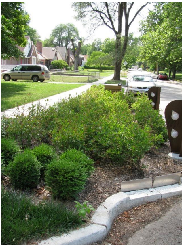
Figure C-11. Outlet of a roadside bioretention pop-out equipped with a V-notch weir for flow monitoring.
