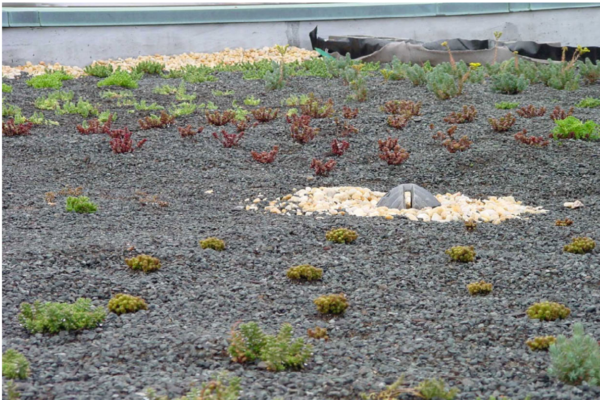
Figure C-8. White gravel indicates a no plant zone for a green roof.
