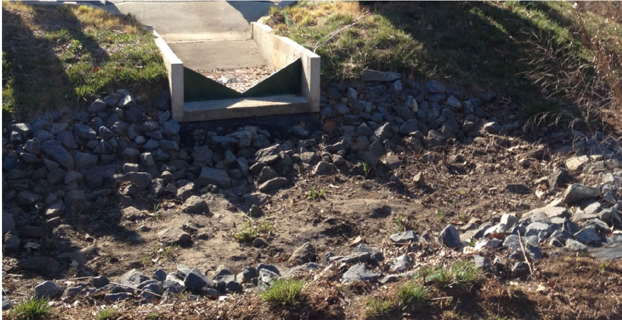
Figure C-10. Inlet curb cut with a v-notch weir.
