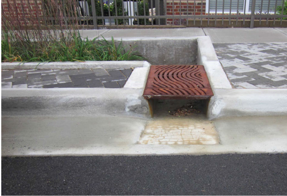
Figure C-2. Inlet sump to remove gross solids.
