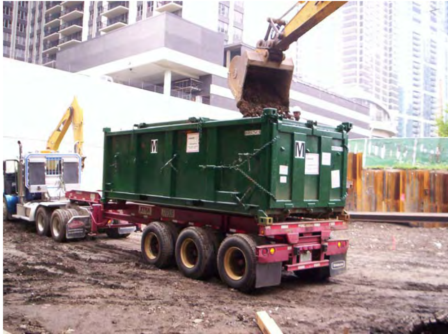
Loading of Impacted Soils
