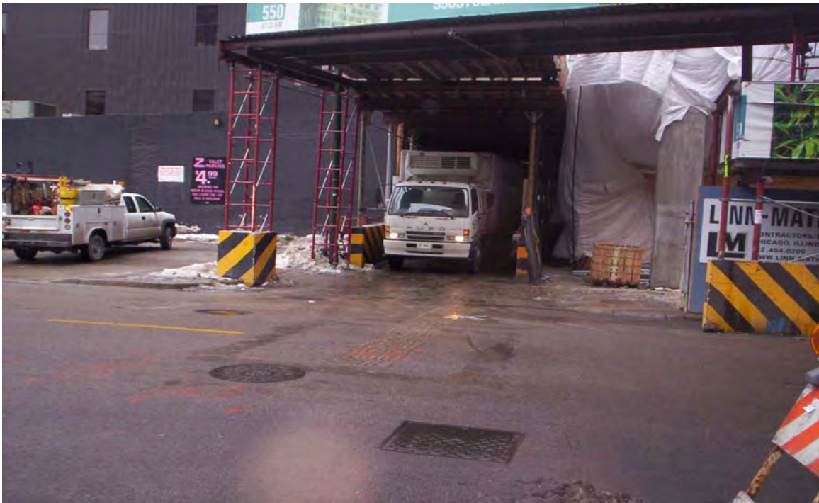
Photo 2: Taken east to west. Shows south end and alley locations of planned test pits prior to beginning work.
