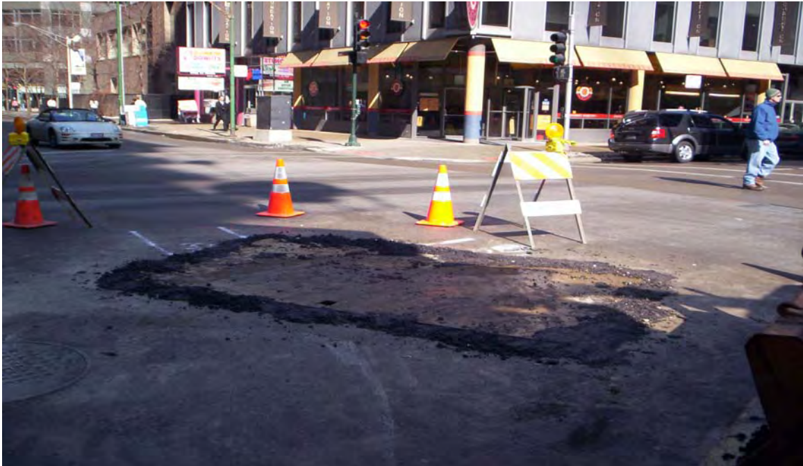
Photo 6: Taken east to west. Shows placement of steel plate over test pit #1 after its completion.
