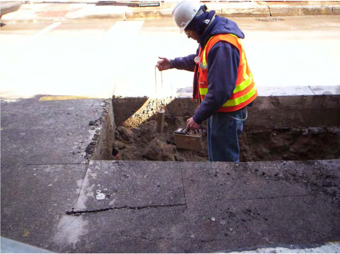
Photo 7: Taken west to east. Shows radiation screening of soil in test pit #2.
