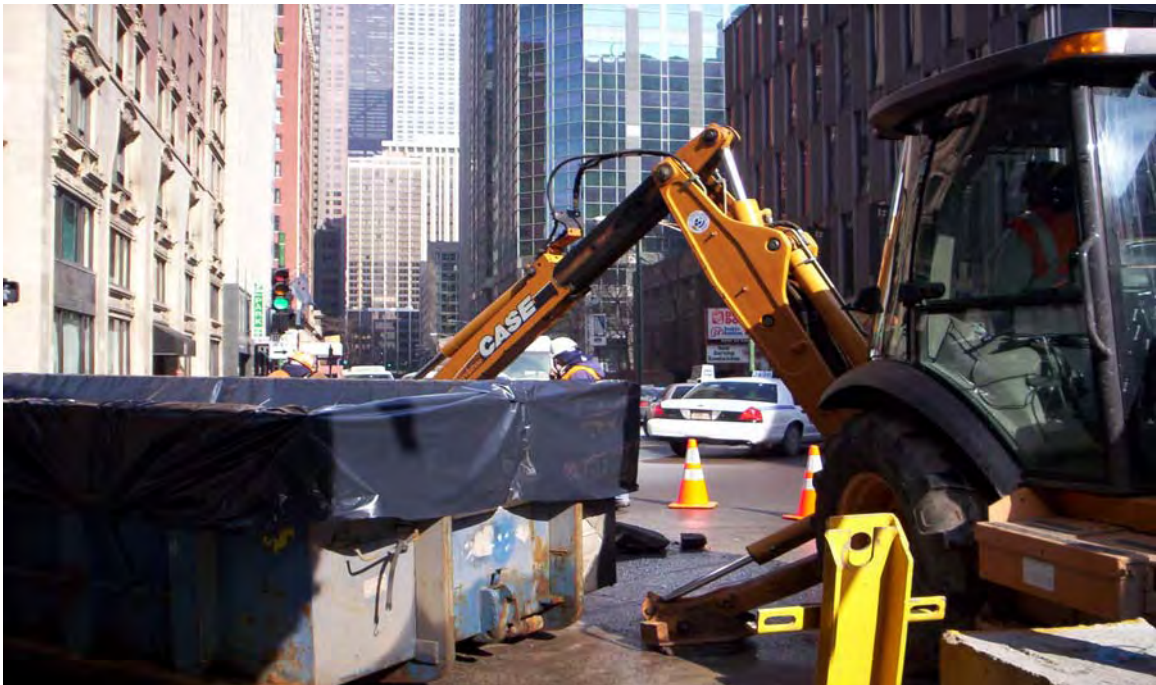
Photo 4: Taken south to north. Shows excavation of test pit #1, with backhoe loading clean soil into roll-off box.
