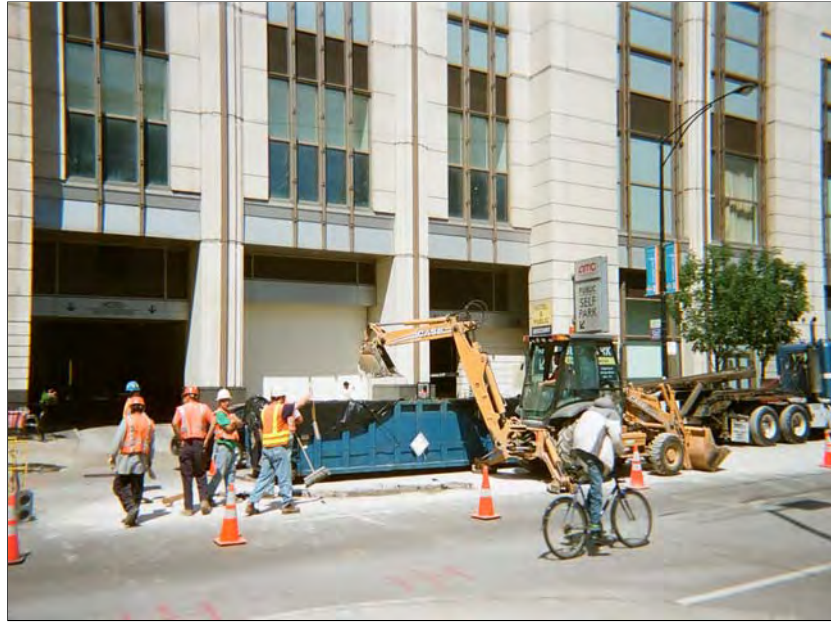
Photo 5: Taken south to north. Screening of trench soils for radiation from the surface during excavation.
