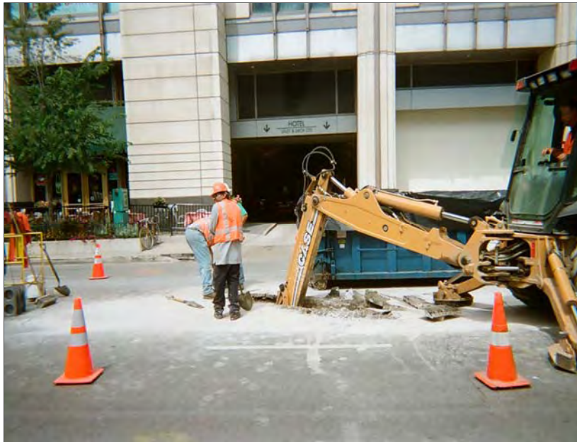
Photo 4: Taken south to north. Beginning of trench excavation using backhoe. Shows narrow width of trench.
