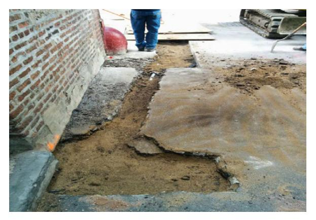
Photograph looking east toward St. Clair Street. Geotextile has been placed in the contaminated portion of trench, conduit installed in trench and a thin layer of sand placed over the geotextile and conduit prior to placement of concrete to complete the installation.
