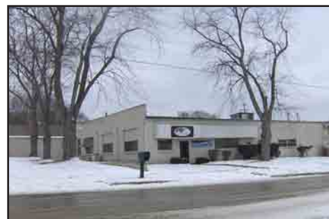
The completed Hi-Tech Flexible Products building.
