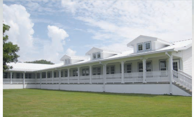
The light-colored roof reflects heat while front windows provide ample daylighting.
