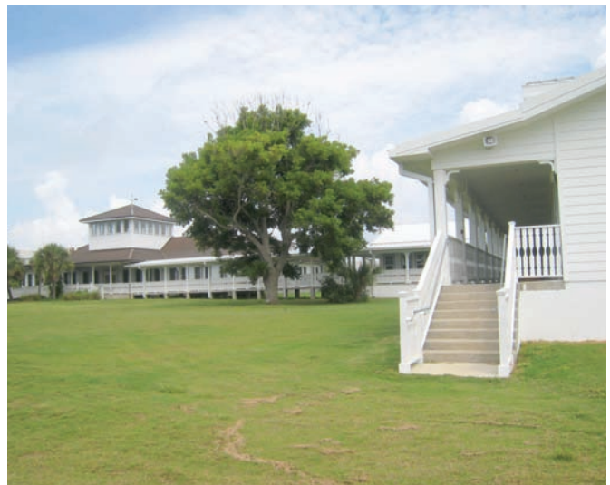
The building's siding is a wood pulp, sand, and cement composite made of recycled material.
