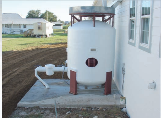
A storage tank collects rainwater from the cistern.
