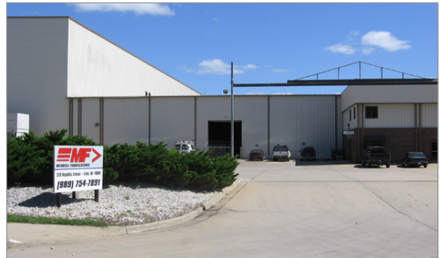
The completed Merrill Fabricators facility.
