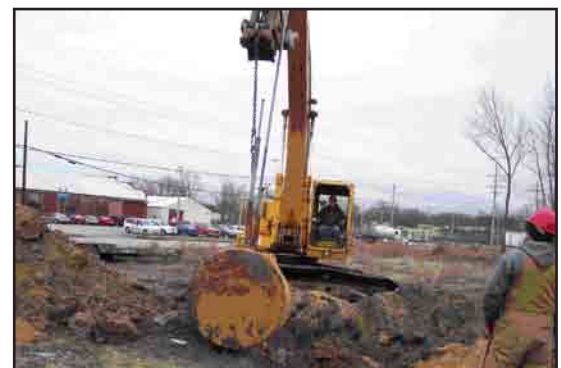
Removal of underground storage tank at former bulk petroleum plant.
