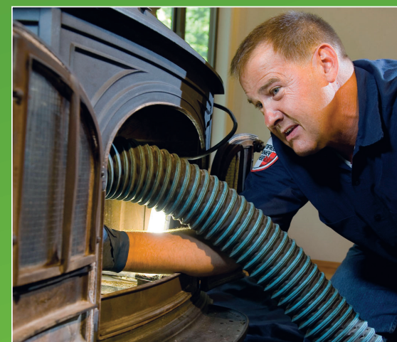
Stoves and chimneys should be inspected by a certified chimney sweep once a year to prevent chimney fires.
