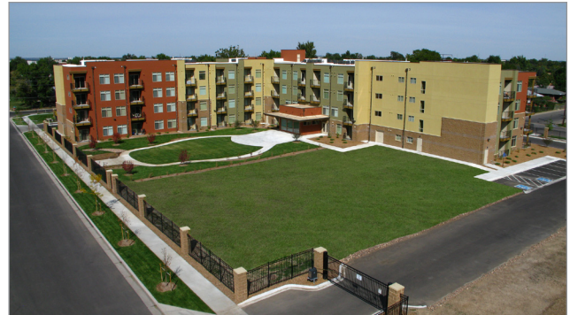
The redeveloped Dahlia Square Senior Apartment complex.
