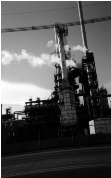
Figure 5: The Conoco Refinery in Commerce City, CO
