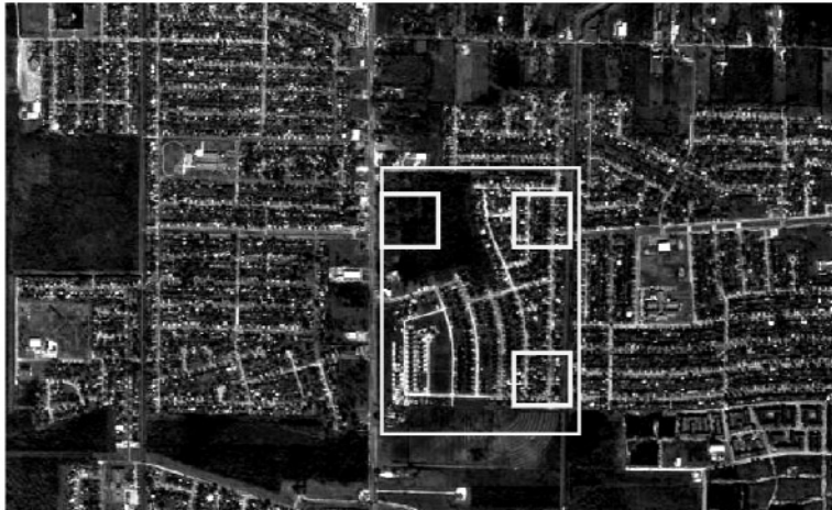
Figure 6: Kennedy Heights Subdivision and Approximate Crude Oil Storage Tank Locations
