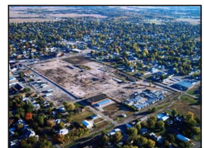
The former International Harvester site, following demolition of remaining structures.
