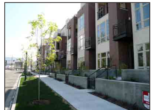
The CitySide Lofts, after redevelopment.
