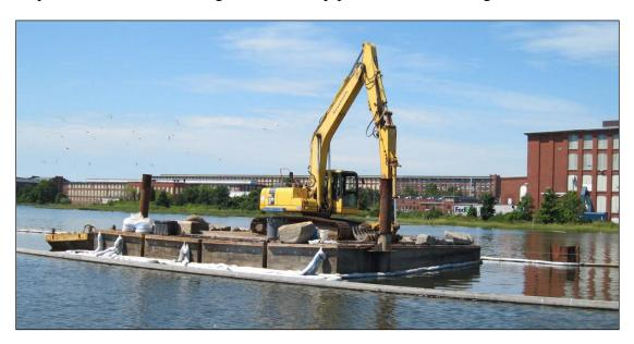
Figure 8. Debris removal excavator and debris storage scow
