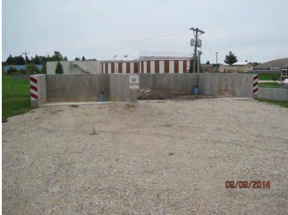
Photo 2: Grit pad used for draining materials derived from sewer cleanout.
