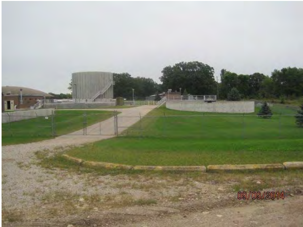
Photo 3: Wastewater treatment plant.
