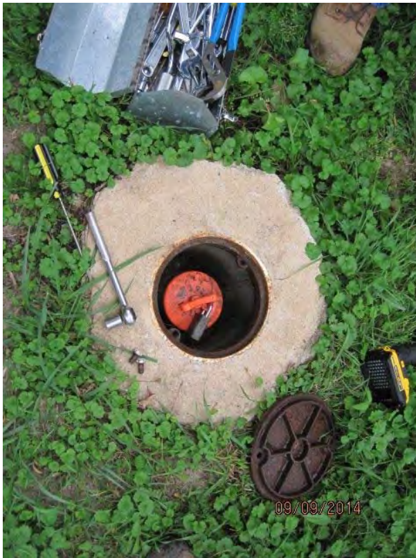
Photo 5: MW-2A showing locking well cap.
