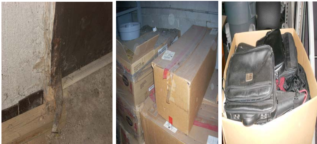
From left: an example of corrosion; dusty and opened boxes; and moldy computer bags. (EPA OIG photos)
