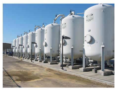
Figure 3-5. Single Pass Ion Exchange System Installed at California Domestic Water Co.
